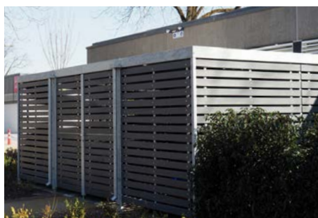
Wanden bekleed met horizontale open belatting in RAL 7011
